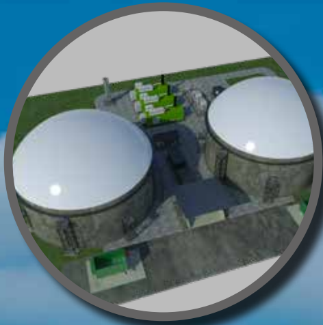
BIOGAS PLANT WITH CONCRETE TANKS
